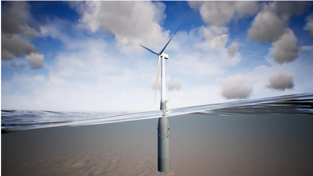
Figure 2. Concept image of a Hywind Tampen floating wind turbine (mooring system not shown).
