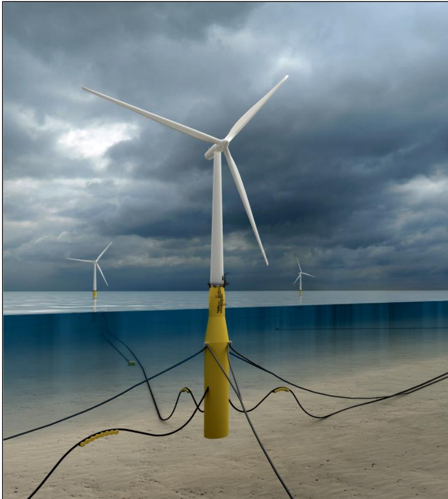
Figure 2. Image of the Hywind floating wind turbine, mooring and power transfer cables.
