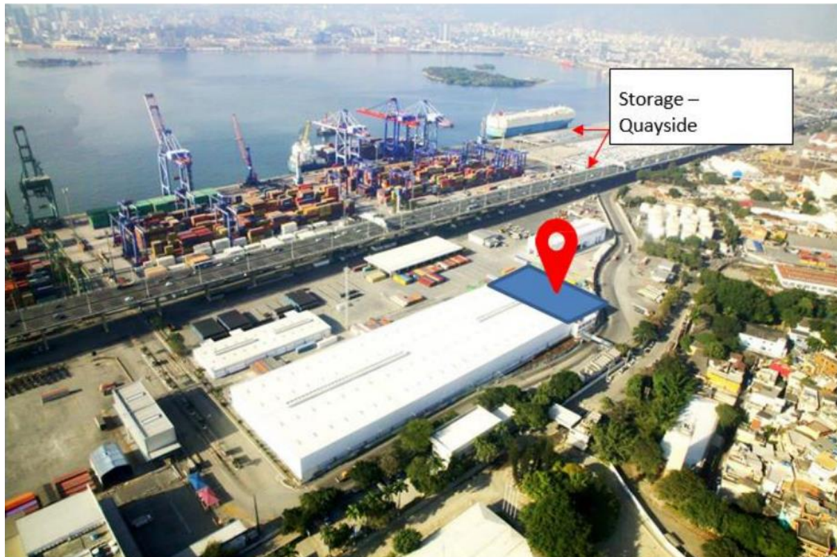
Figure 3-4 Capping stack storage and short access to the Quayside at the port of Rio de Janeiro.
