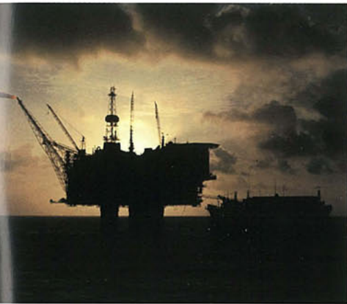
The Statfjord A produces crude oil now, and will also produce gas later.
