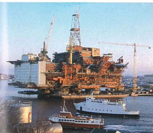
The Statfjord B deck under construction in Stavanger.
