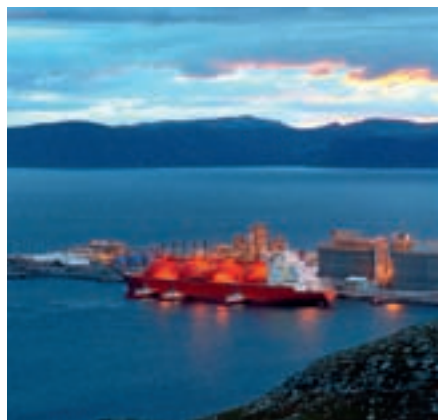
The Snøhvit plant is a pioneering technology project.
