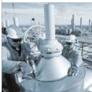
Completing the new facilities at Kårstø.
