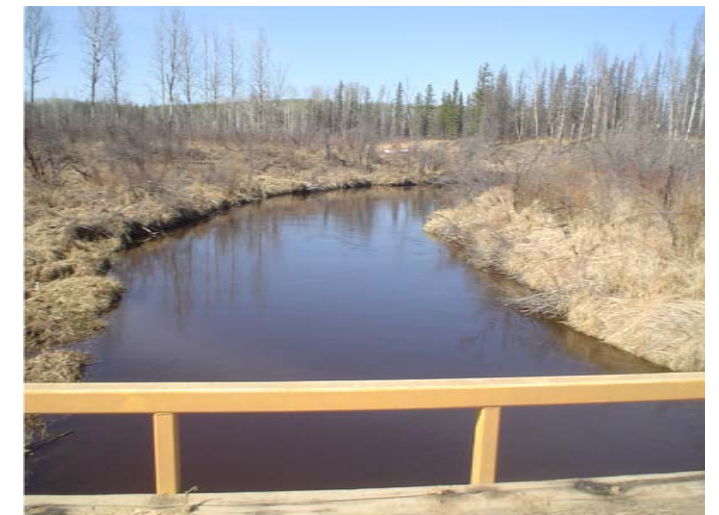
PHOTO 3. View of the bridge crossing on the May River at WCL13.
