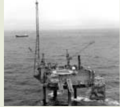
Siri is the first field on the Danish continental shelf where gas is not flared. In addition, almost all the produced water is injected into the reservoir. Following a trial period, the systems for reusing gas and injecting water were put into normal operation in August.
