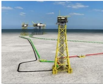
Unmanned Wellhead Platform (UWP TM )
