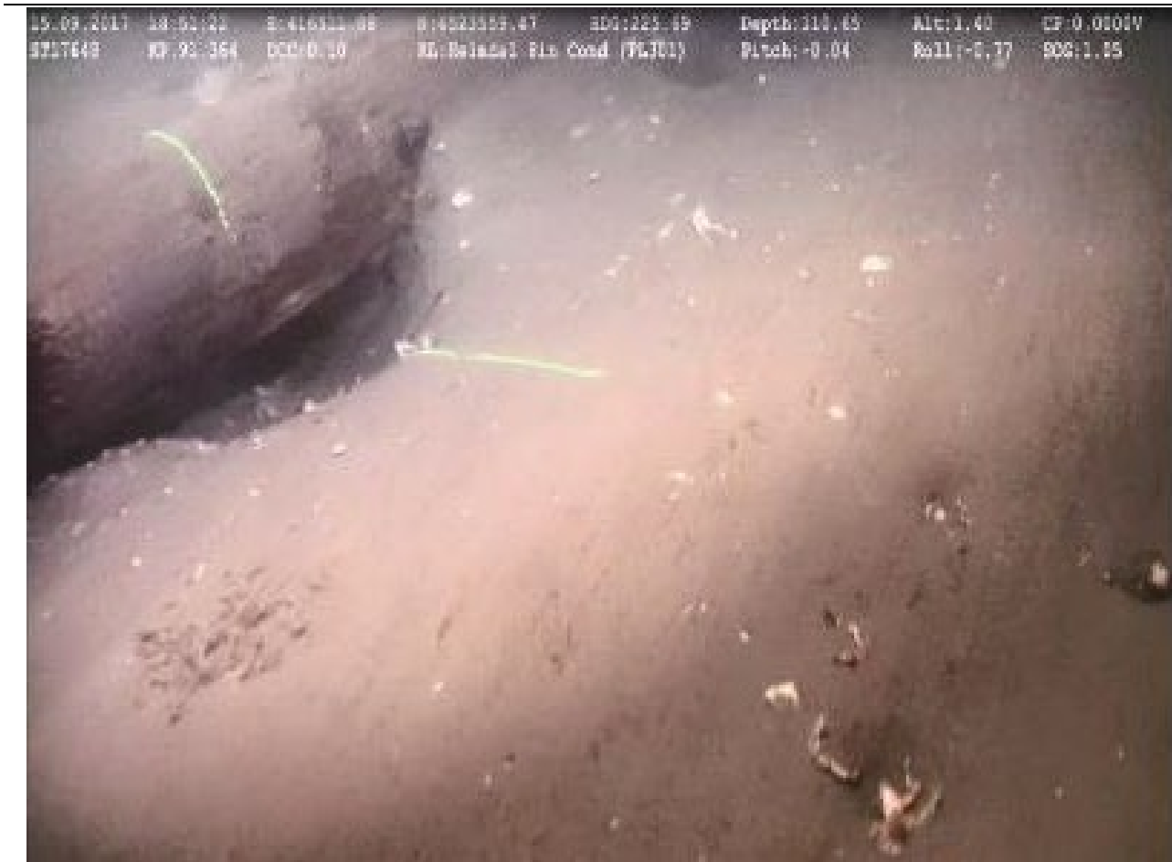
Figure C-4 Image from 2017 pipeline survey at KP 91.364 showing section of PL301 naturally backfilling within the trench
