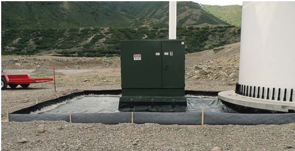
Figure 3.15: Secondary Containment
