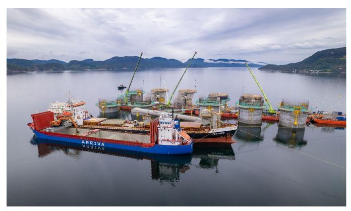
Slipforming at Dommersnes in July 2021, of substructures for Hywind Tampen floating offshore wind farm.
