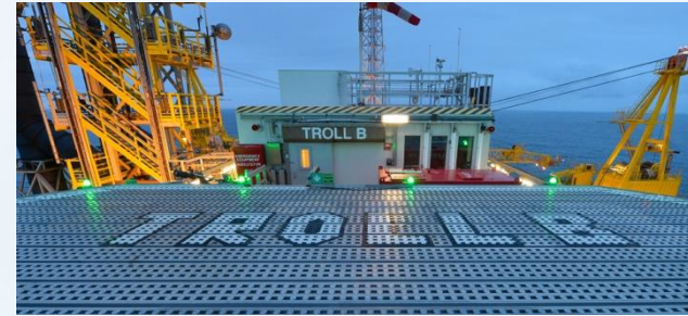
Electrification of the Troll field
