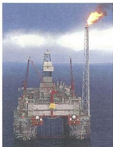
The Heidrun platform in the Norwegian Sea came on stream during the autumn.
