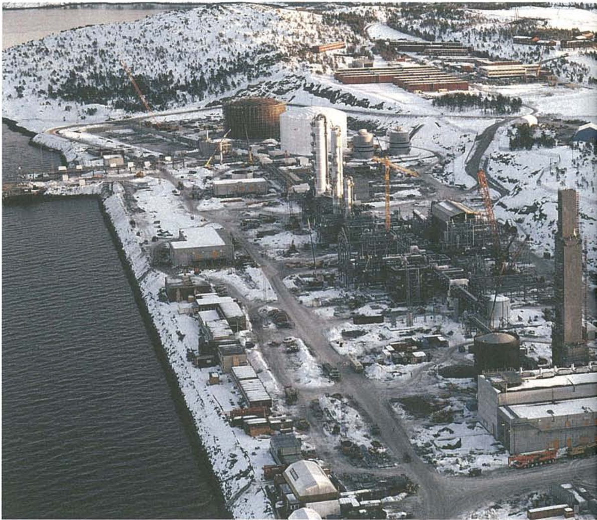
A methanol plant based on gas from the Heidrun field is being built by Statoil at Tjeldbergodden in mid-Norway.
