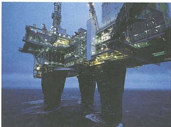
Commissioning the Troll A platform to produce from the North Sea's largest gas field.
