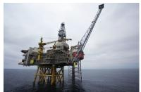
Topsides installed on steel jacket on Valemon field in North Sea
