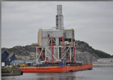
Low pressure production module load-out
