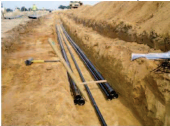
Figure 1.5-4 Duct installation during construction (open cut trench)
