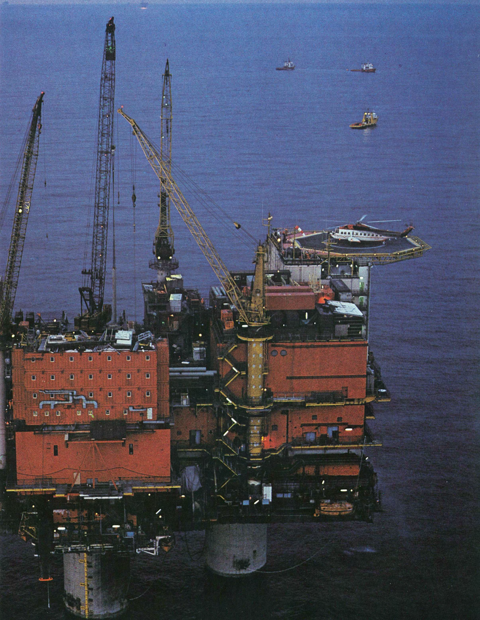
The Statfjord A platform under construction, out on the field.
