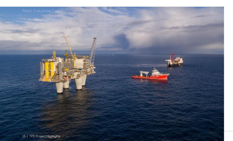
Next plateau extender of Troll gas production which prolongs the field life beyond 2050. Two subsea templates and eight production wells. A new 36" inch pipeline to Troll A and a new process module on Troll A.
