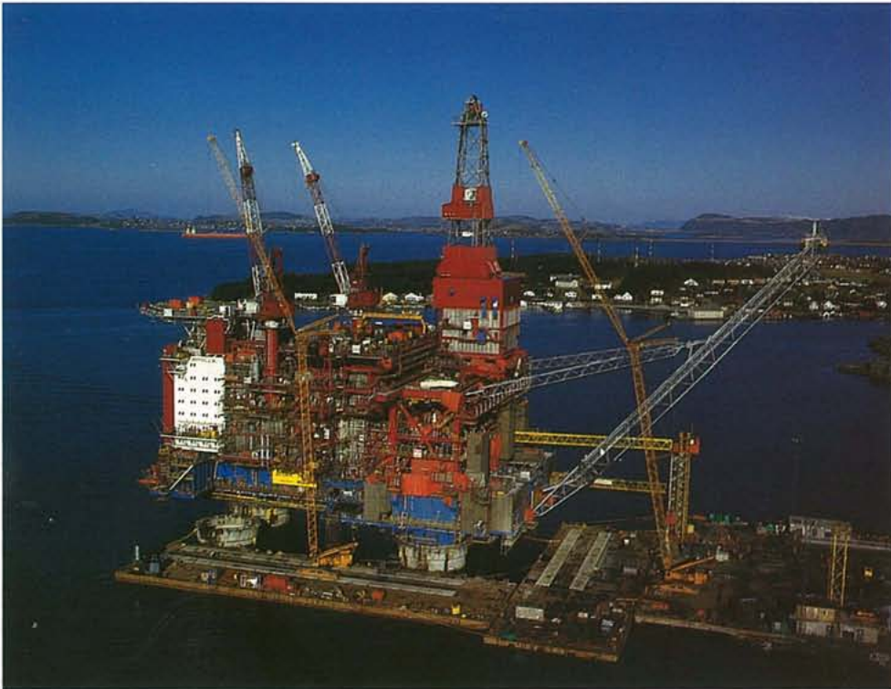
The Gullfaks B deck under construction at Rosenberg Shipyard in Stavanger.
