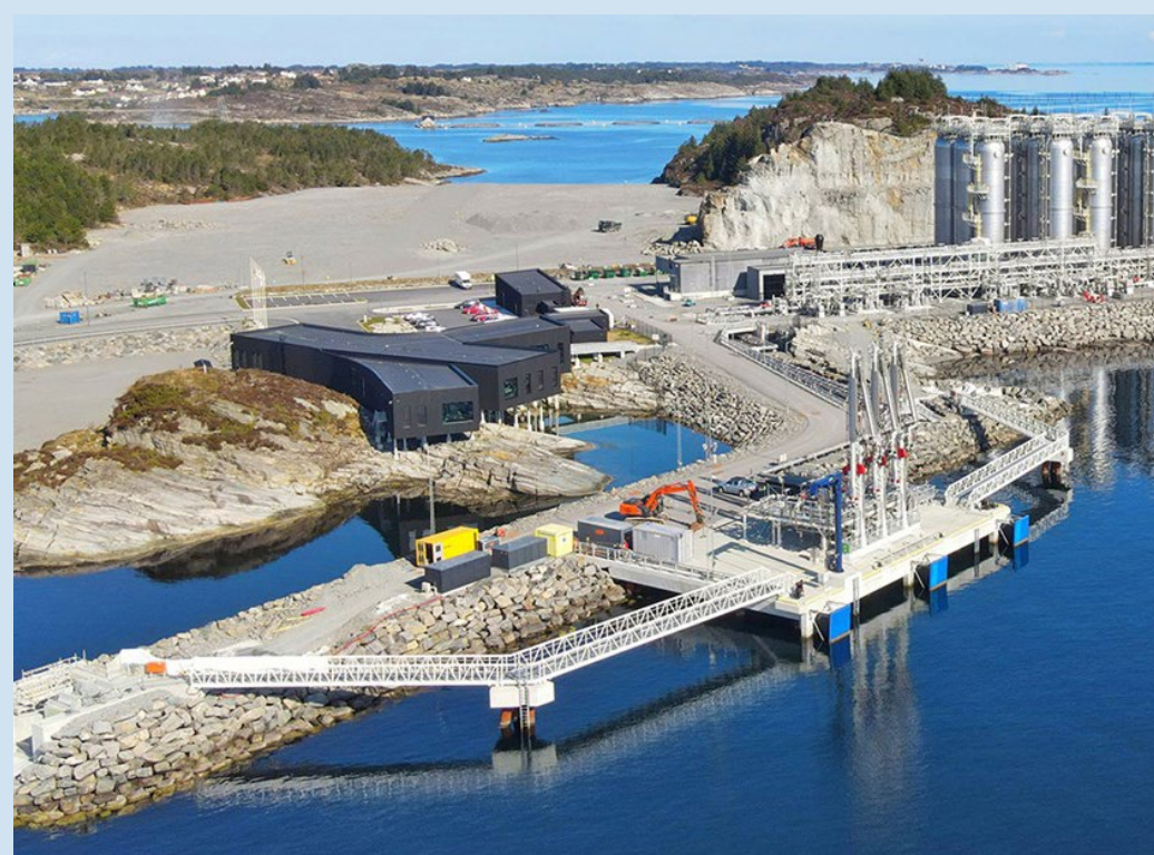
The Northern Lights receiving terminal at Øygarden outside of Bergen, Norway.
