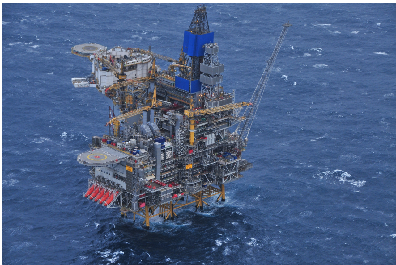
Figure 2.1 Mariner A production, drilling and quarters (PDQ) platform with NLN drilling derrick (blue) cantilevered over the drilling deck
