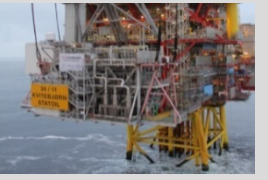
Kvitebjørn compressor installed
