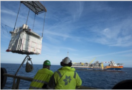
Topside module installed
