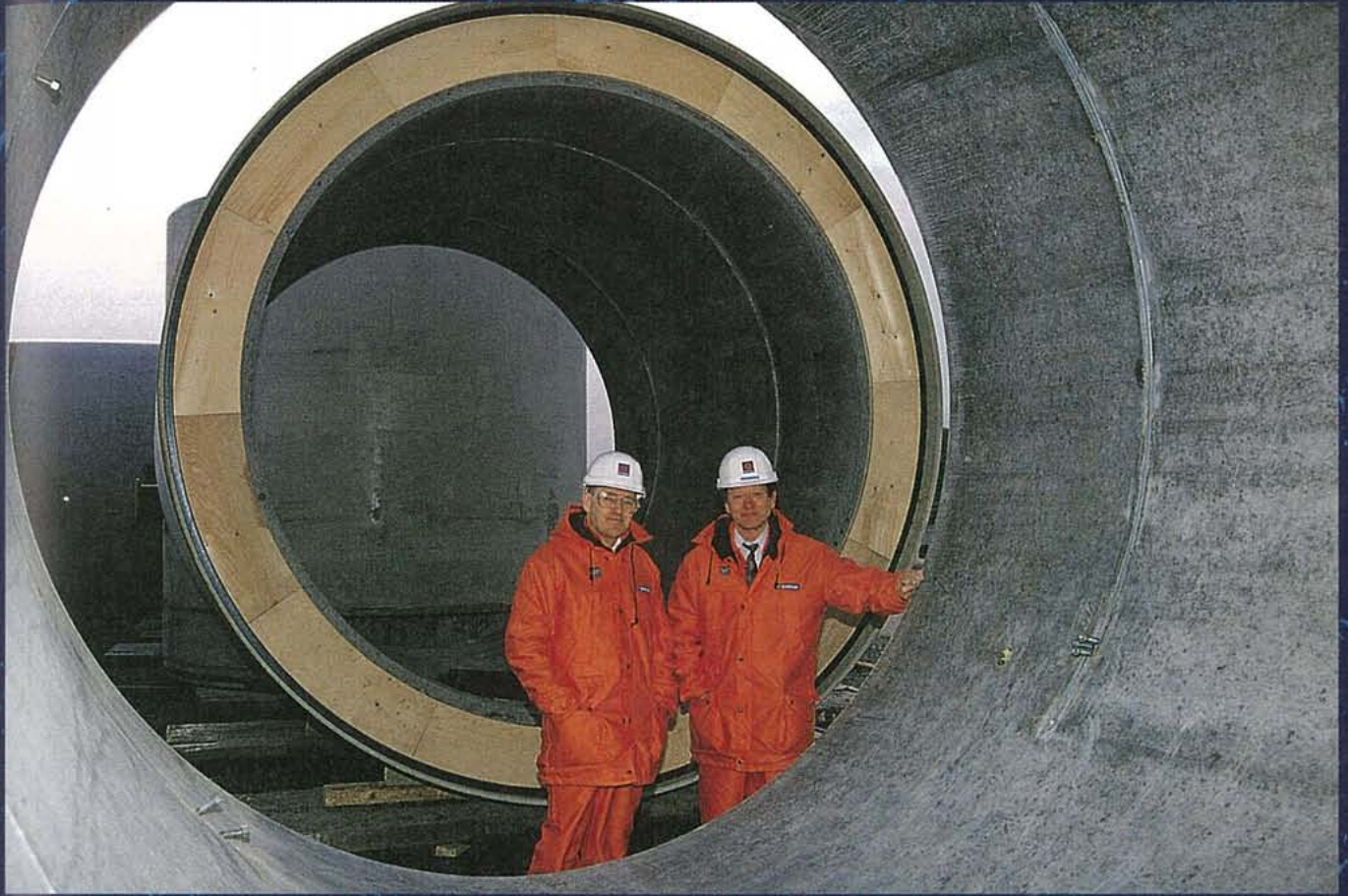
The concrete pipes being used to line the tunnel which will carry Europipe under Lower Saxony's protected coastal wetlands have an internal diameter of three metres - big enough to accommodate two gas pipelines.
