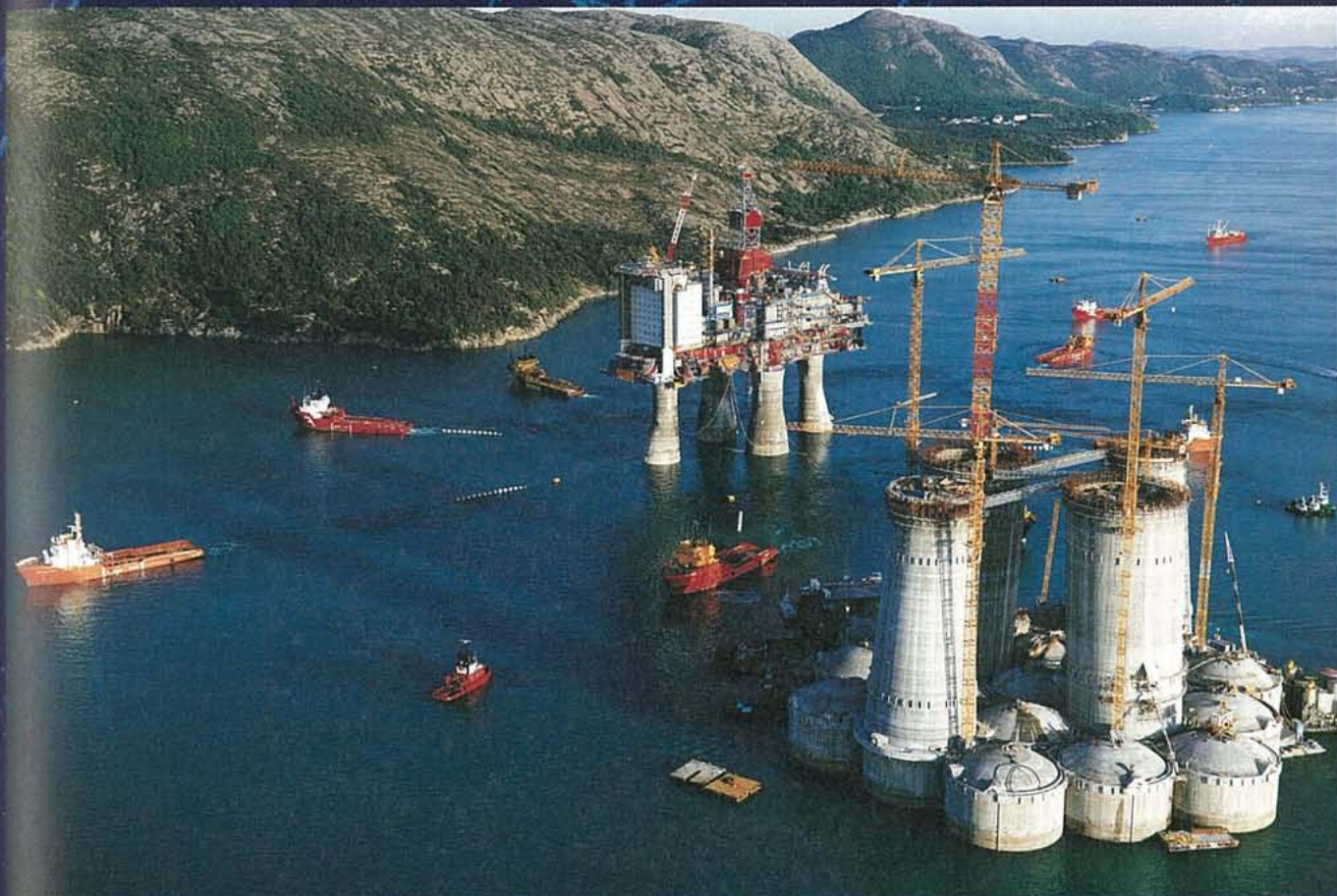
The Sleipner A production platform was towed offshore in early June 1993. Its route from the Cands Fjord outside Stavanger took it past the concrete gravity base structure for another Norwegian gas platform - Troll Gas. This unit is the tallest of its kind in the world.
