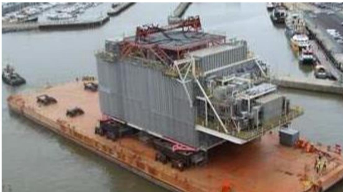
A HVDC module will be integrated in module U00 located on the west side of the weather deck on the Riser Platform.
