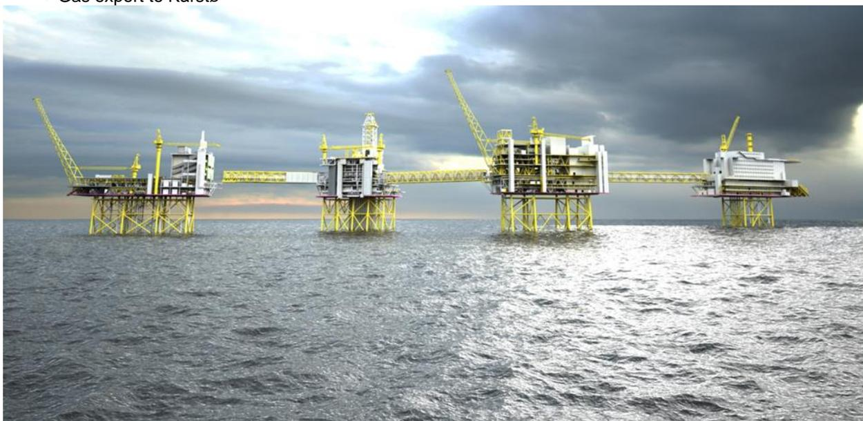
The Johan Sverdrup production facilities will use significant amount of energy in the form of mechanical power and heat. Rotating power is primarily needed for pumps and compressors while the main consumer of heat is the oil stabilization process.
