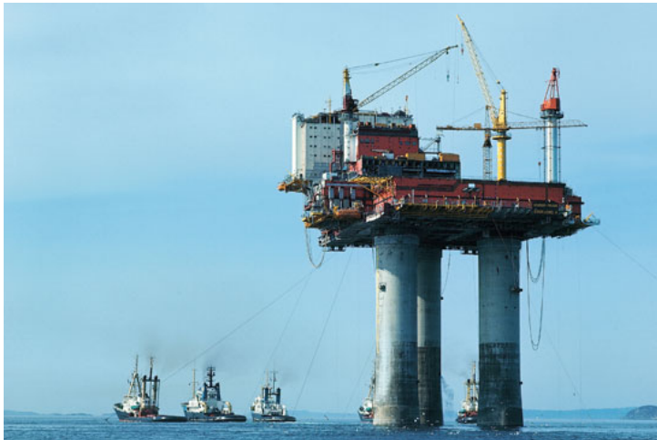
Figure 5. From towing of Statfjord A prior to installation.
