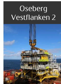
Ongoing Unmanned Wellhead Platform (UWP™)
