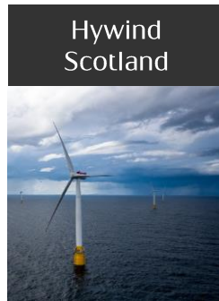
In operation Offshore floating wind
