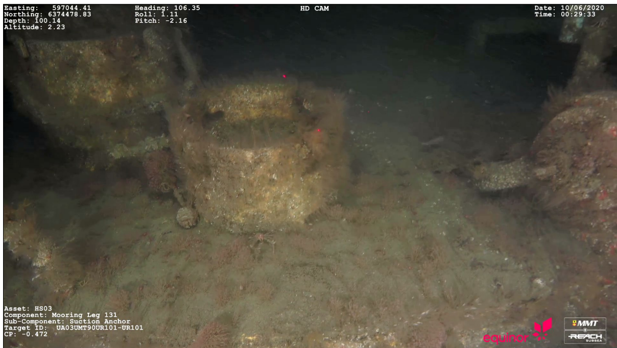
Figure 8 Example image from the top of the Suction Anchor (HS03 – Suction Anchor 131).
