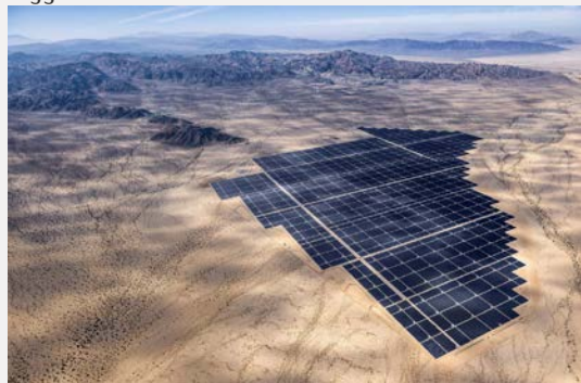
The 550 MW Desert Sunlight solar PV power plant in California's Mojave desert - reportedly the biggest in the world
